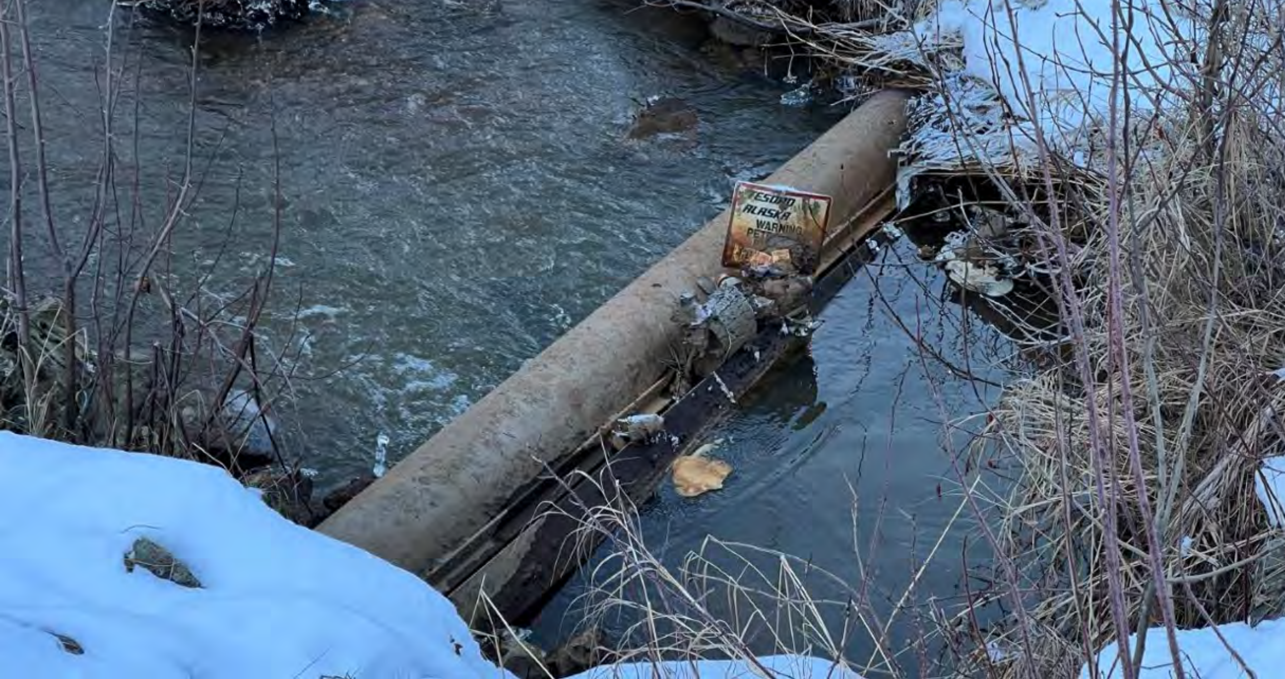
The pipeline facility going across Fish Creek near the preferred alignment of the proposed trail.
