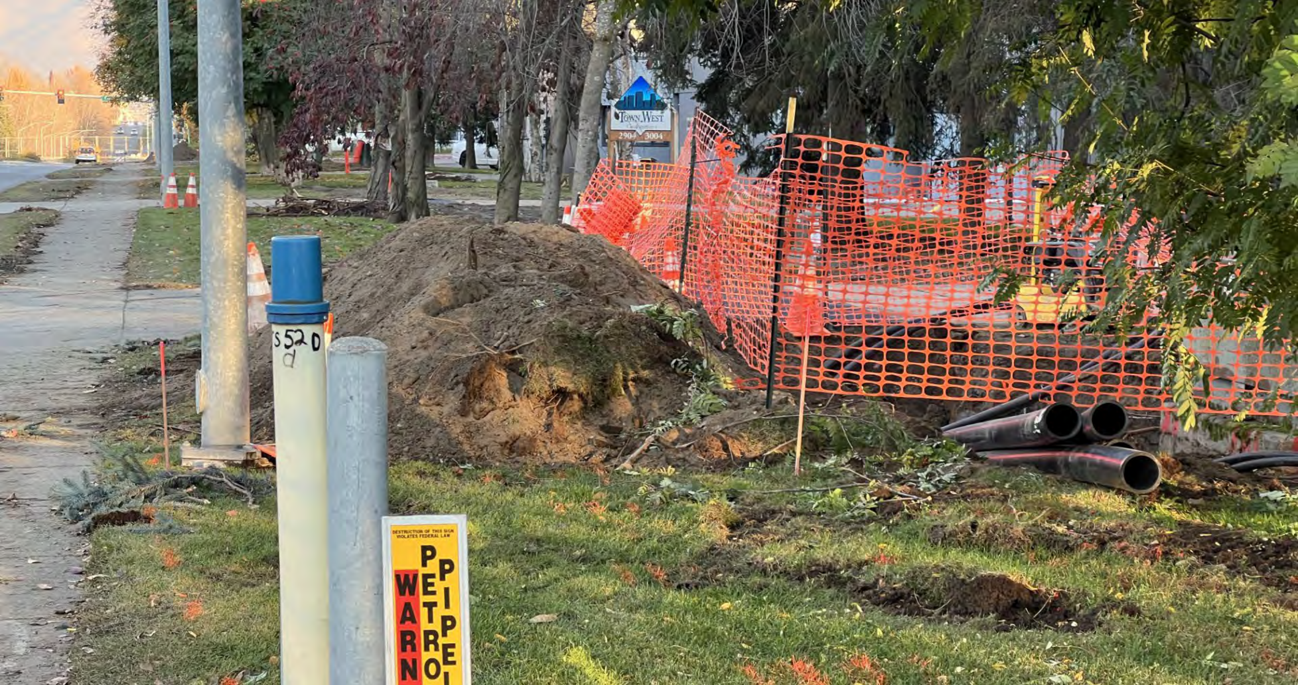
Similar infrastructure projects near pipelines have been completed successfully without incidents . 2024 Utility Work on Northern Lights Blvd.
